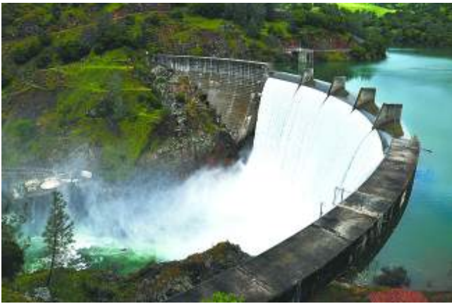
Water spilling over the dam at Englebright dam in April 2011.
